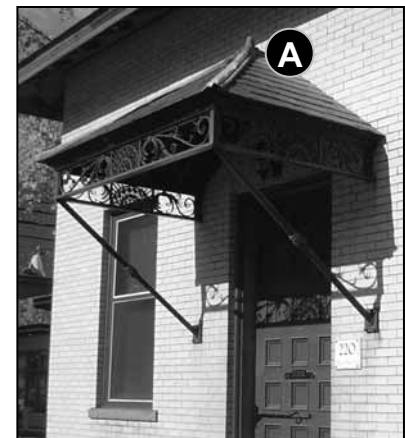
Fig. 5-40: 220 Main St. Intricate metal roof design.
