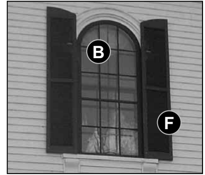
Fig. 5-16: 213 Main St. Custom wood storm windows and working shutters match the design and blend nicely with the historic architecture.
