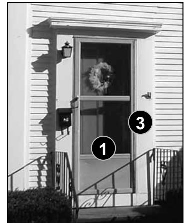
Fig. 5-14: 102 Jefferson St. The bare aluminum storm door here would blend in with the architecture of the doorway more if it were recessed slightly, and painted.
