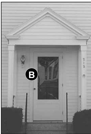
Fig. 5-13: 213 Washington St. The painted wood storm door on this entry blends in with the entry design.
