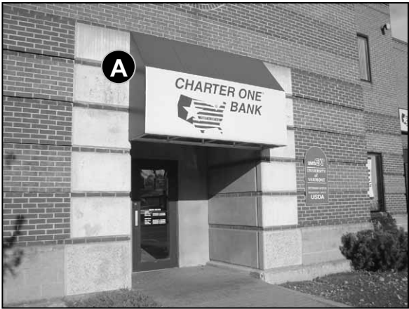
Fig. 5-94: 338 Main St. Simple details like the concrete cornerstones at this entry help to evoke earlier design styles.
