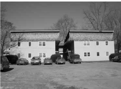
Photos: 400 Main Street on the corner of Putnam Square (top); parking near School Street and Pleasant Street (middle); residential apartments at 326 Pleasant Street (bottom).
