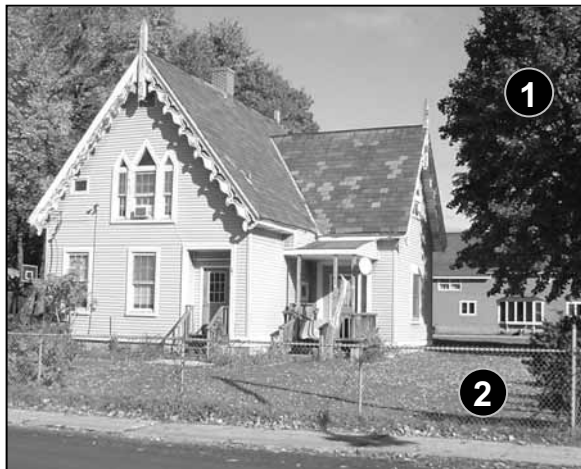
Fig. 5-59: 207 Depot St. The chain link fence here does not match the character of the house. A wooden picket fence would be more appropriate.
