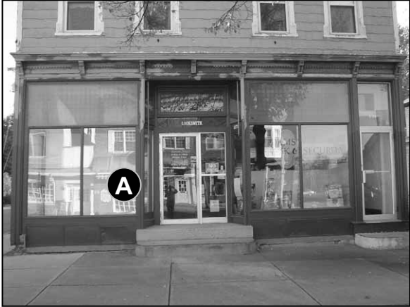
Fig. 5-79: 497 Main St. Original storefront still exists.
