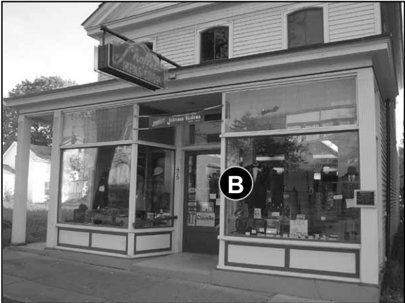
Fig. 5-80: 475 Main St. Original storefront design has been preserved.
