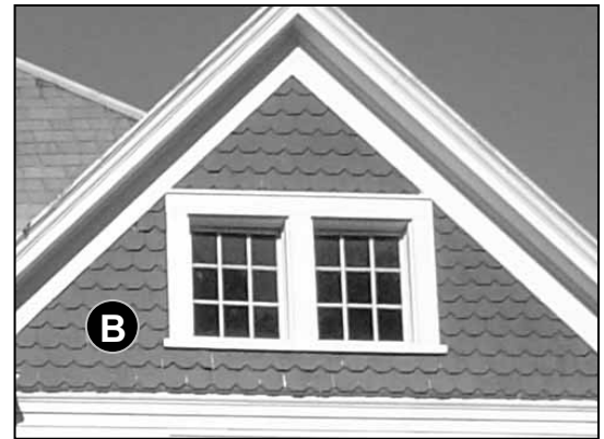
Fig. 5-31: 206 Main St. Original scalloped shingles are used only on the gable ends of this home to give them a more unique appearance.
