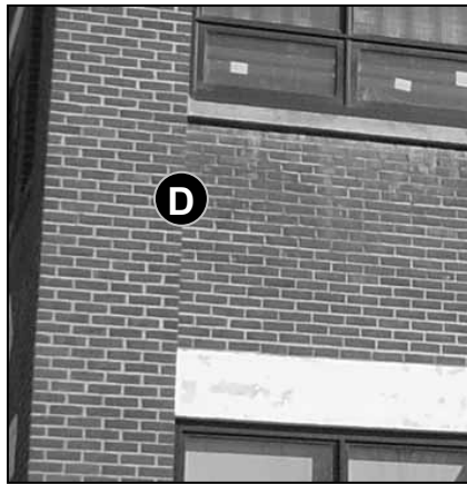
Fig. 5-33: When cleaning masonry surfaces, avoid using harsh or abrasive cleaning agents that can permanently discolor the surface.
